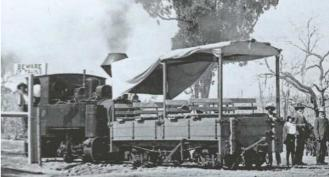
A real wagon converted to carry an Inspection Party along the railway during the construction phase.
